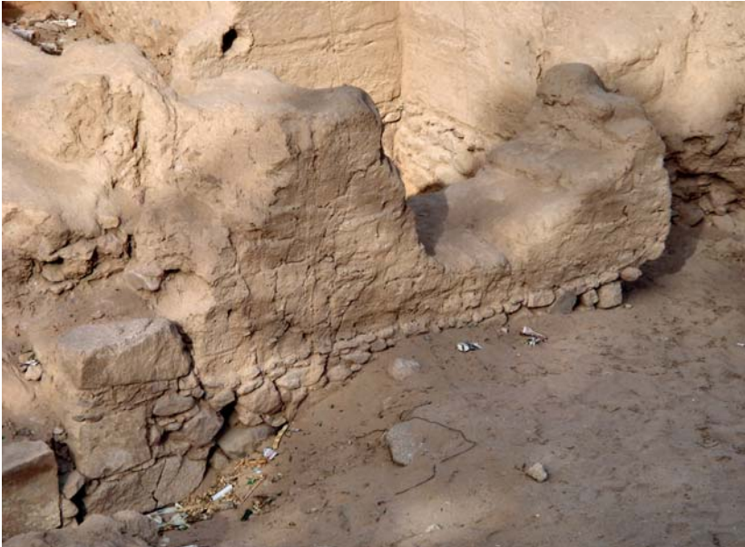
Fig. 9: Architecture from Byzantine Ailana. Note use of a few foundation courses in stone, which were topped by a mud brick superstructure (photo by K. Damgaard).
